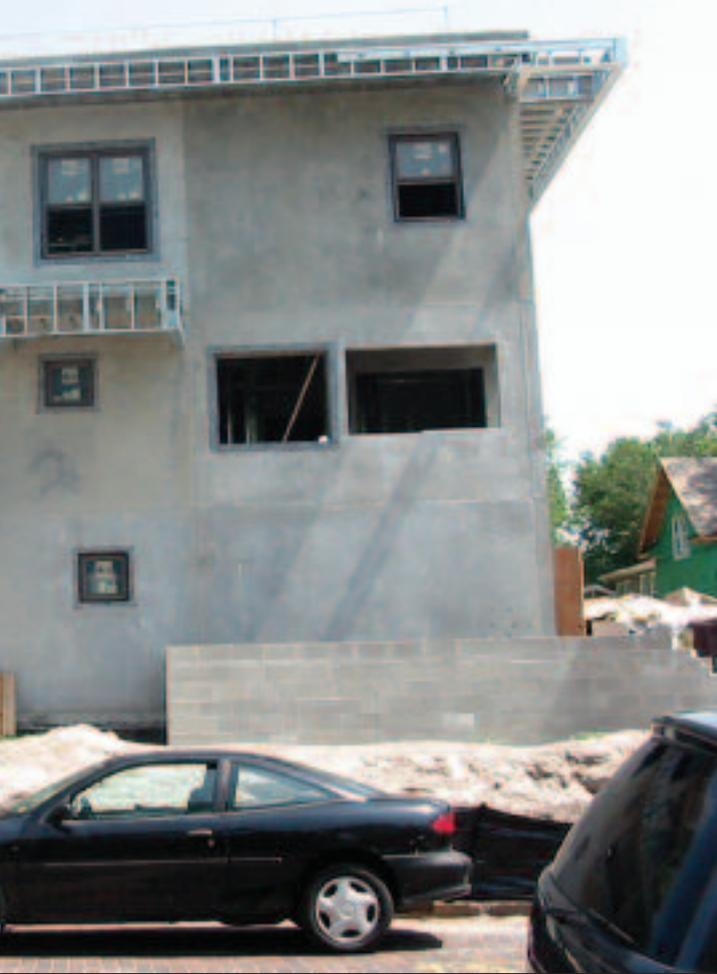
Left: Precast concrete sandwich walls created a secure and airtight panelized system. Below: Concrete balconies and precast overhangs provide shade and, on the third floor, contribute to the rain-water harvesting system. Photos: Jim Niehoff
