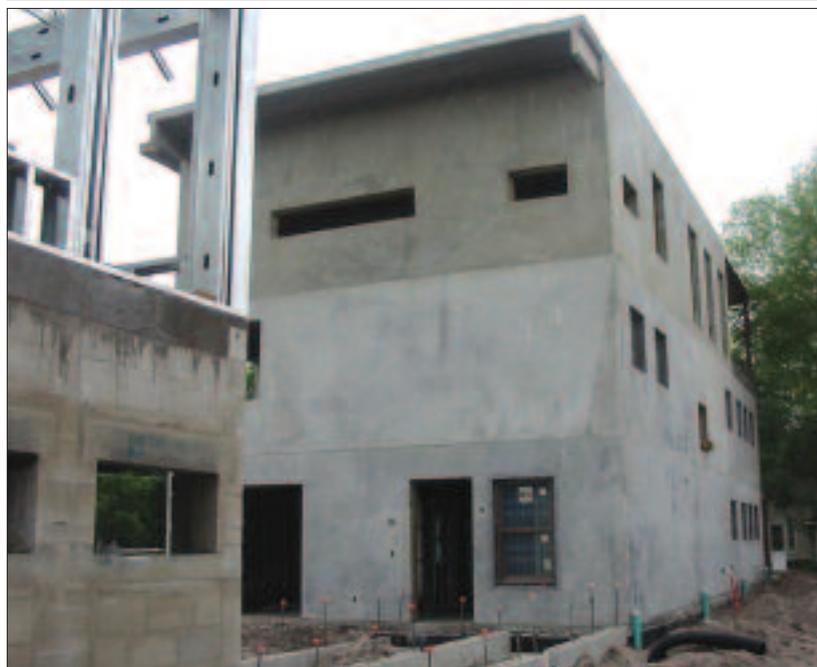
Left: The first floor of the garage was built with concrete masonry units, while the additional living suite employed a steel frame. Above: Special attention was given to the openings for windows and other penetrations to maintain airtightness and energy efficiency.
